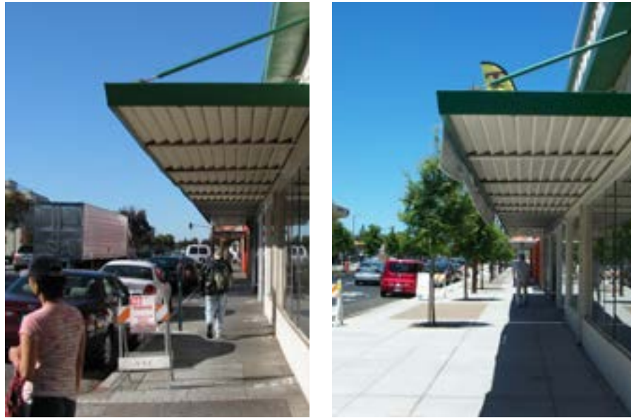
EL CAMINO REAL, 700 BLOCK (BEFORE AND AFTER)
