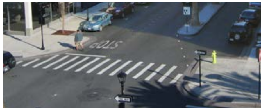
SIDEWALK “BULBOUTS” AND “CONTINENTAL” CROSSWALKS
