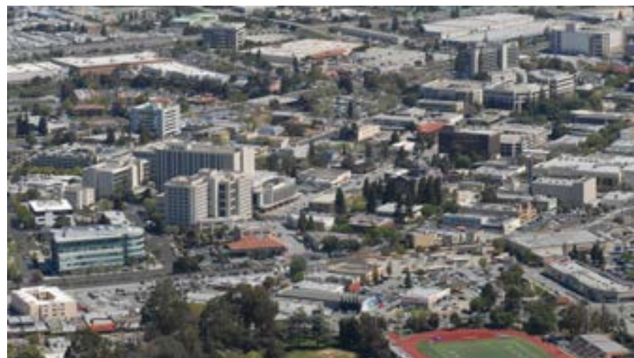
LACK OF COHESION IN BUILDING HEIGHTS
