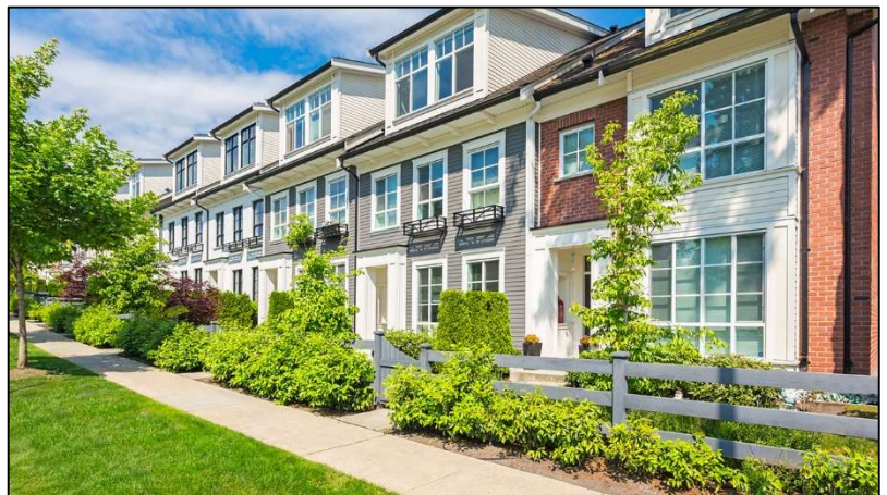
Entrances to individual units facing the street
