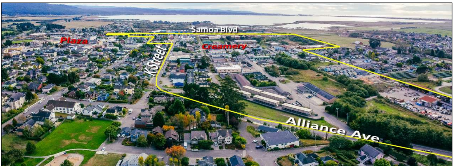
The Gateway Area Boundary, looking south (see Figure 1 for more detail).
